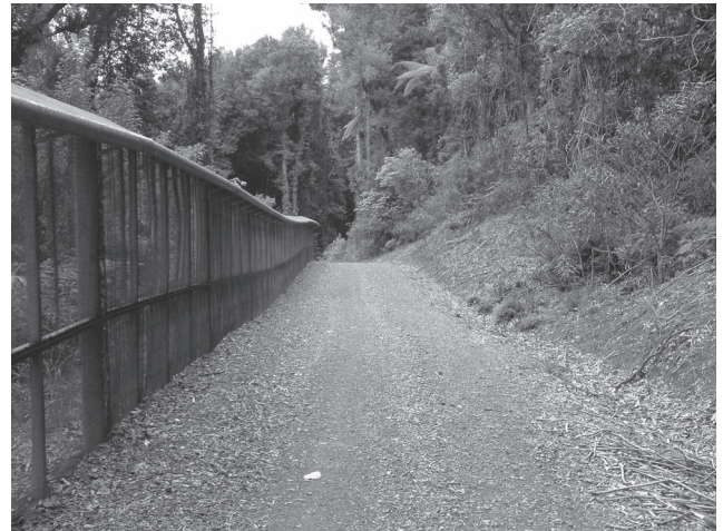
Fig. 1. Exterior view of the Xcluder 'Kiwi' pest-proof fence at Maungatautari, with gravel service road to the right.
